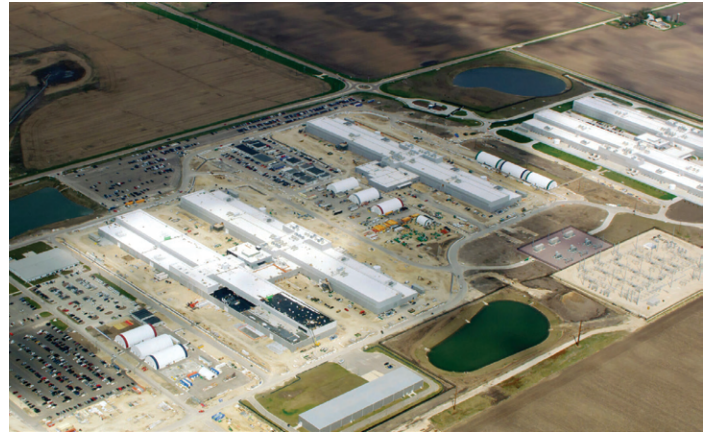
▲ Gurler Road Data Center DeKalb, Illinois
