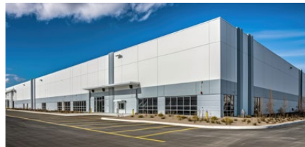
Bridge Point I-55 Commerce Center – Building 2, Romeoville Projected Completion Q3 2025 RBA: 172,042 SF. 172,042 SF available
