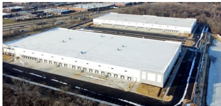
1100 Tollgate Road, Elgin Completed Q1 2024 RBA: 248,400 SF. 248,400 SF available
