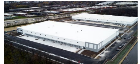
1120 Tollgate Road, Elgin Completed Q4 2023 RBA: 189,530 SF. 189,530 SF available
