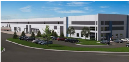
320 Overland Drive, North Aurora Completed Q4 2023 RBA: 408,195 SF. 408,195 SF available
