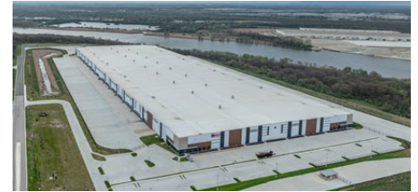
2903 Schweitzer Road, Joliet Completed Q4 2023 RBA: 977,145 SF. 977,145 SF available
