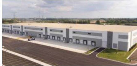
1191 E. Main Street, East Dundee Completed Q3 2023 RBA: 175,905 SF. 175,905 SF available
